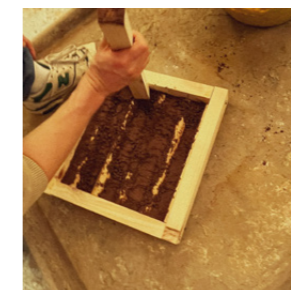
Process of mixing rammed earth mixture and compressing it into the CNC milled formwork
